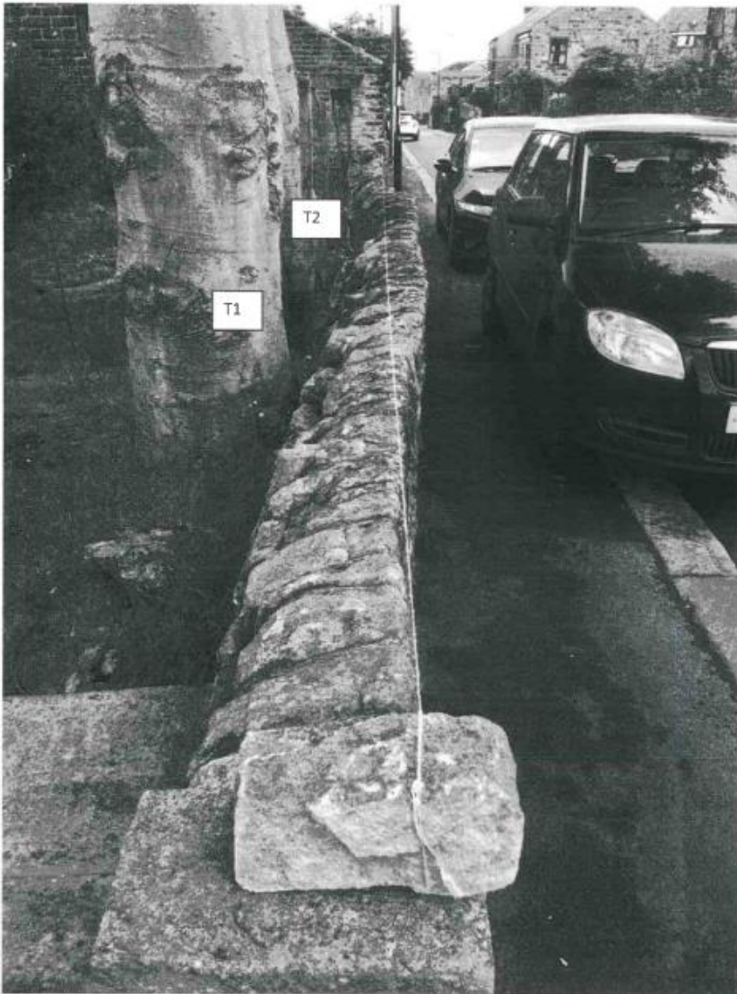
Figure 1 Wall position looking south along Middle Lane
