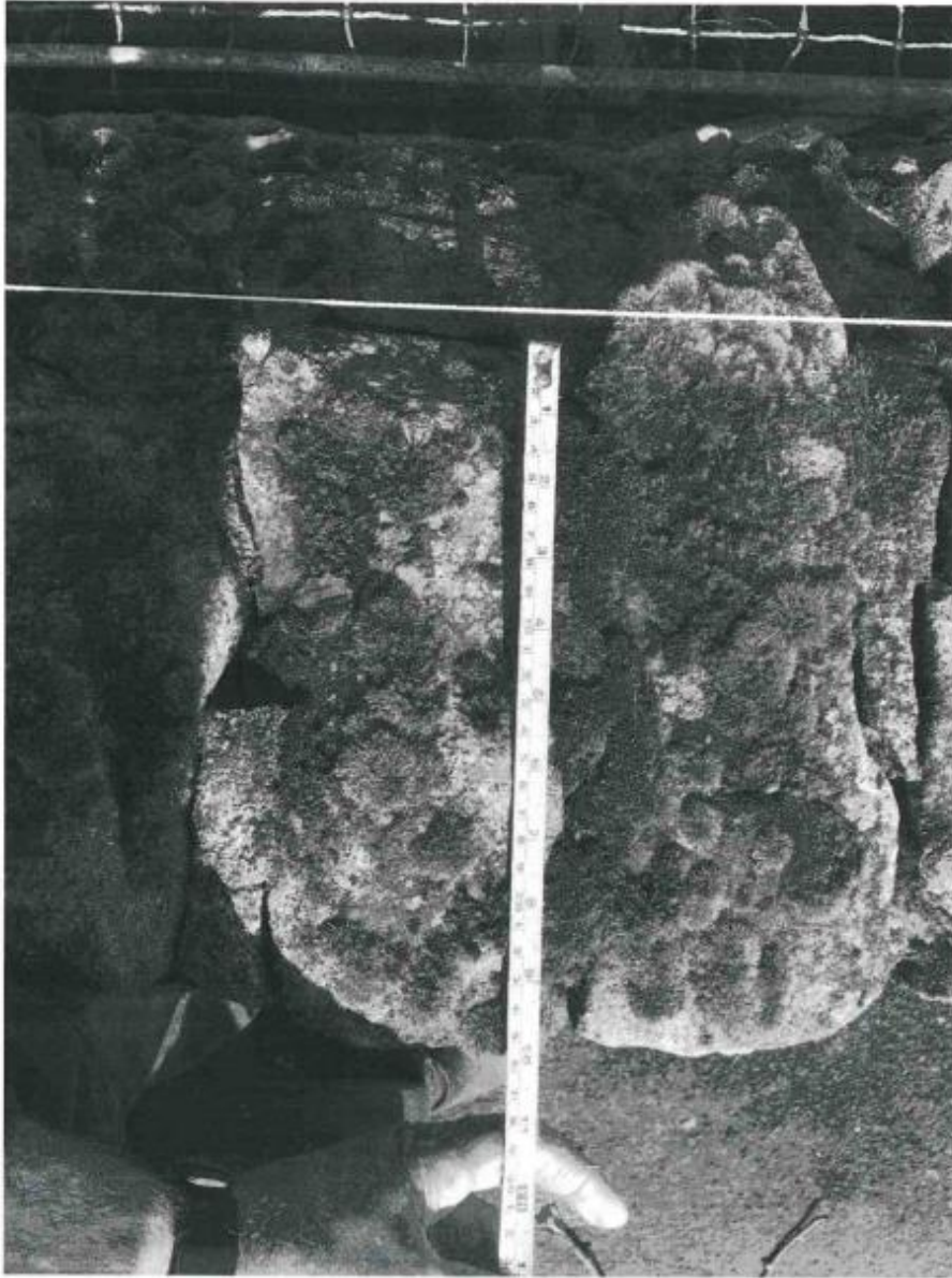
Figure 2 Measurement of wall position relative to original wall line
